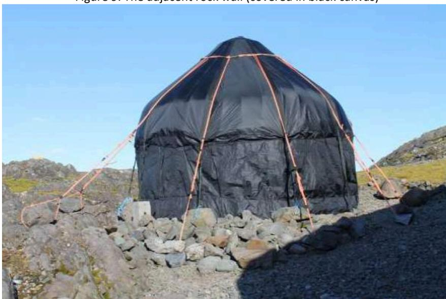
Figure 10. The final result, including the 10+10 ties to the ground.
